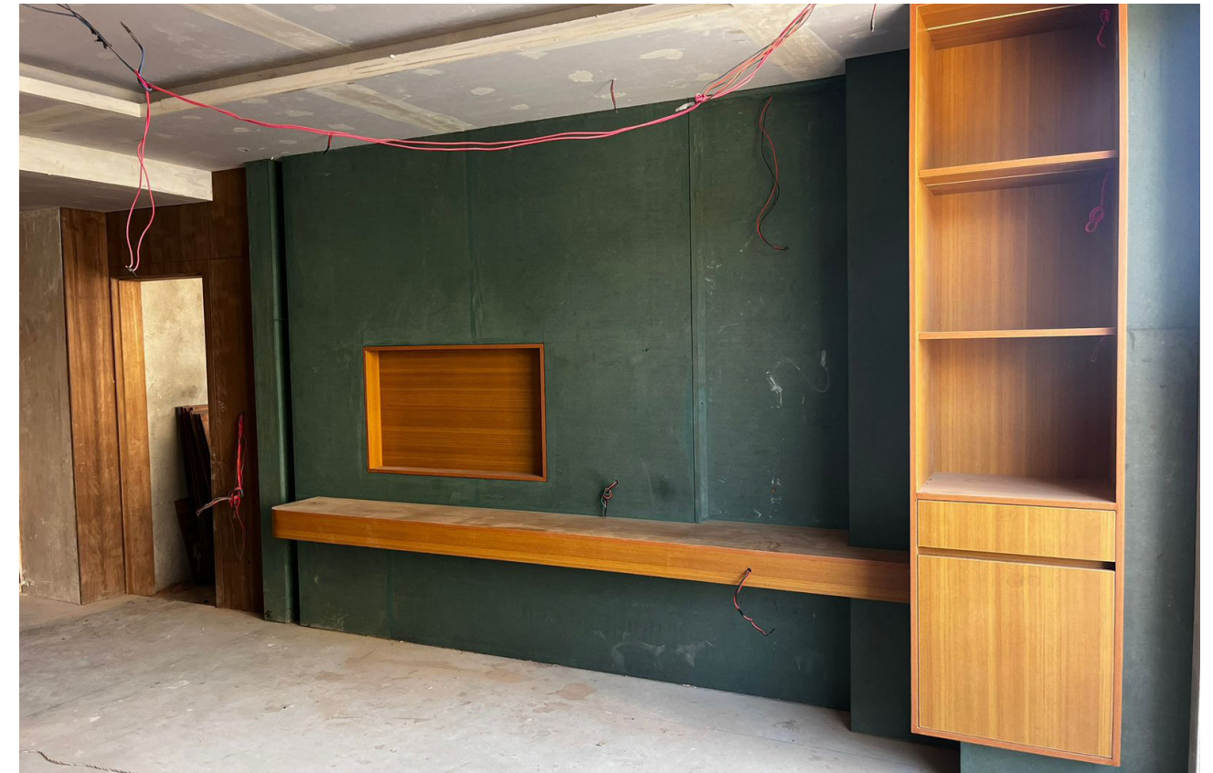
Figure: Construction phase showing Interior of TV Shelf and Cabinet
