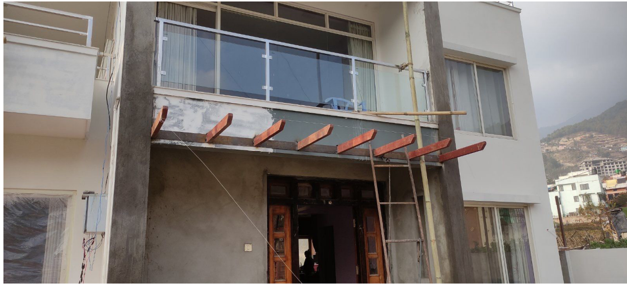
Figure: Image during construction of site
