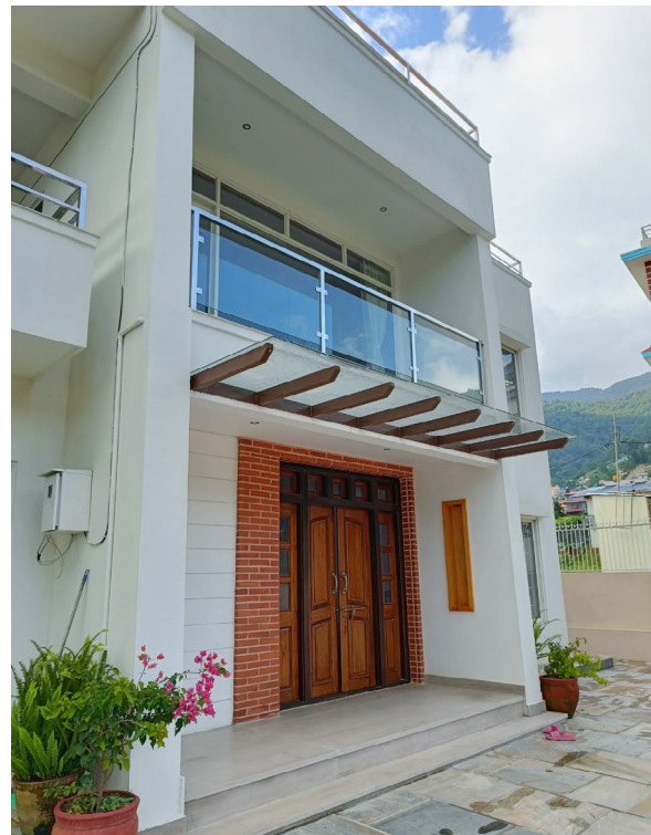
Figure: Final Image after construction and finishing
