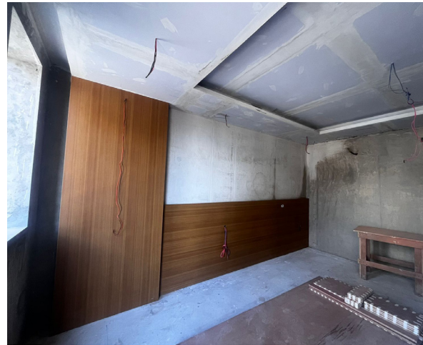
Figure: Construction phase showing wood veneer panelling in the wall.
